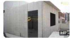
Transforming Spaces: Penthouse Construction Revealed 676 views · 5 months ago
